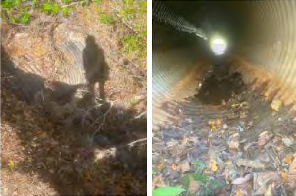
**Location 13:** water overflow to wetland and sidewalk undermining. Install 12" deep x 6" wide footing on upstream side of sidewalk to deter undermining and restore area with sod. Finish grade of grass on outfall side is to be 1/2" below the existing sidewalk grade to prohibit blockage of runoff.
