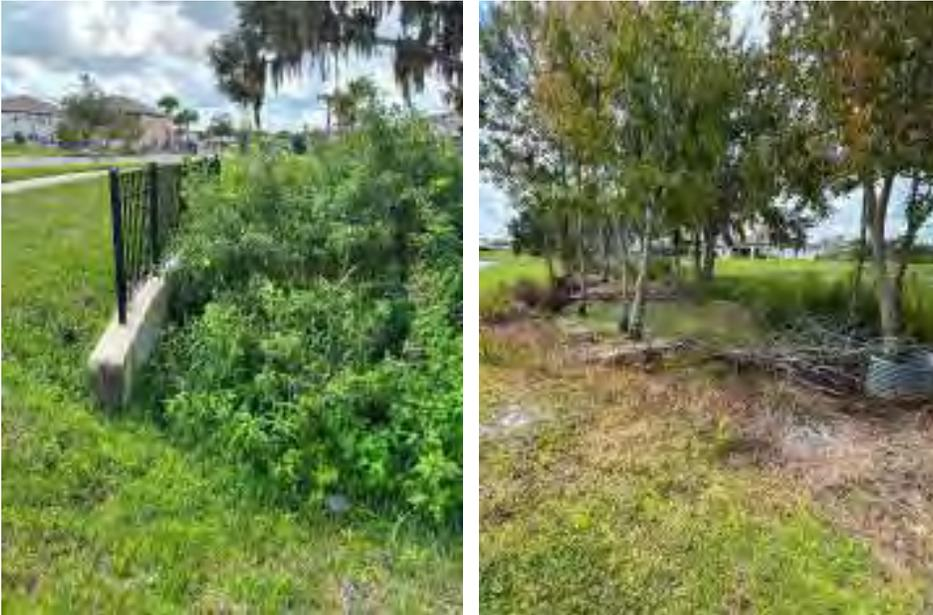
**Location 11:** Overgrown vegetation has blocked the end of the mitered end section and is prohibiting the proper flow/discharge from the pipe. Remove overgrown vegetation 5' around MES to provide for proper flow.
