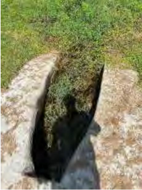
**Location 13:** Mitered End Sections (MES). MES is showing signs of erosion and is being undermined. Erosion observed beneath existing mitered end section. Add #57 stone with compacted fill beneath mitered end section to prevent future erosion and undermining. Place filter fabric and rip rap extending 2' minimum out from existing structure to stabilize the area around the existing mitered end section. Sod disturbed areas. Refer to Key Map for specific location.
