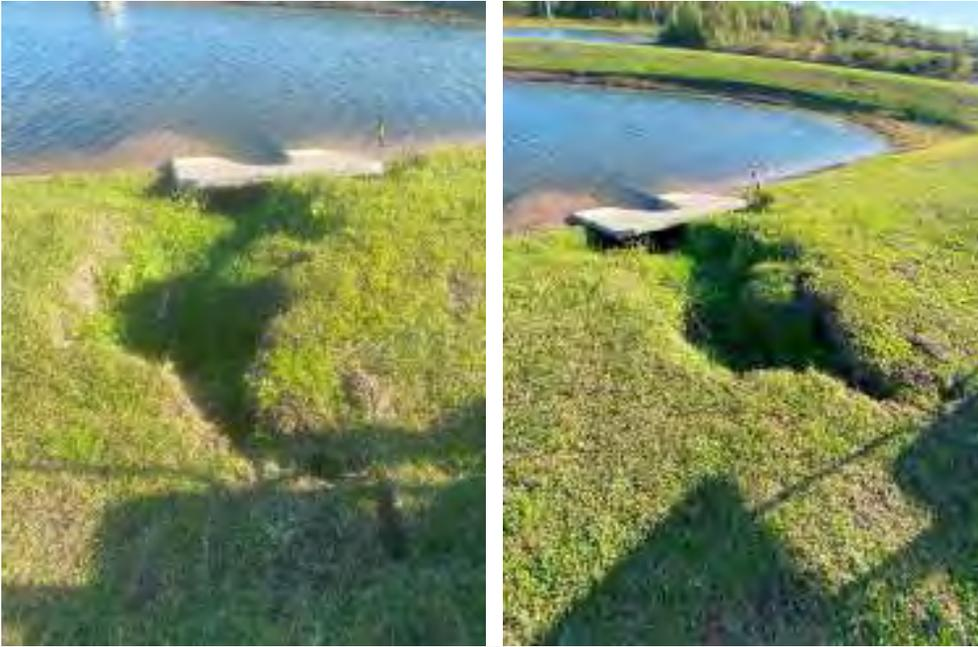
**Location 4:** Erosion caused by concentrated water flow from between the houses and fluctuation of water levels. Install approximately 120 LF flexamat along eroded pond bank.
