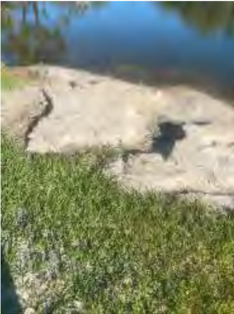
**Location 9:** Erosion of pond bank due to concentrated flows from between houses. Repair with flexamat. Sod all disturbed areas.
