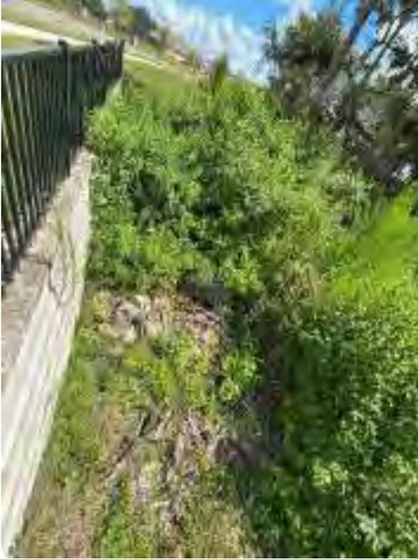
**Location 8:** Overgrown vegetation needs to be cleared 5' from headwall to allow proper flow and discharge into and from drainage pipes.
