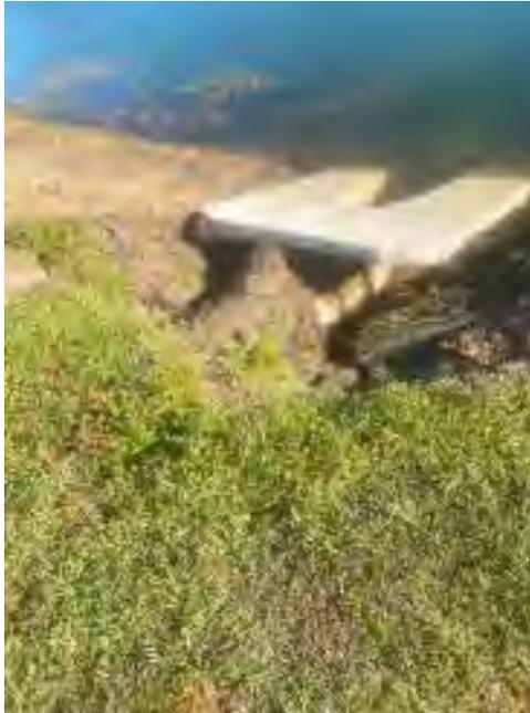
**Location 2:** Homeowner pool drain is discharging onto CDD property causing the grass to die and area to erode. Request homeowner to discharge pool drain on residents' property to eliminate erosion of CDD property.
