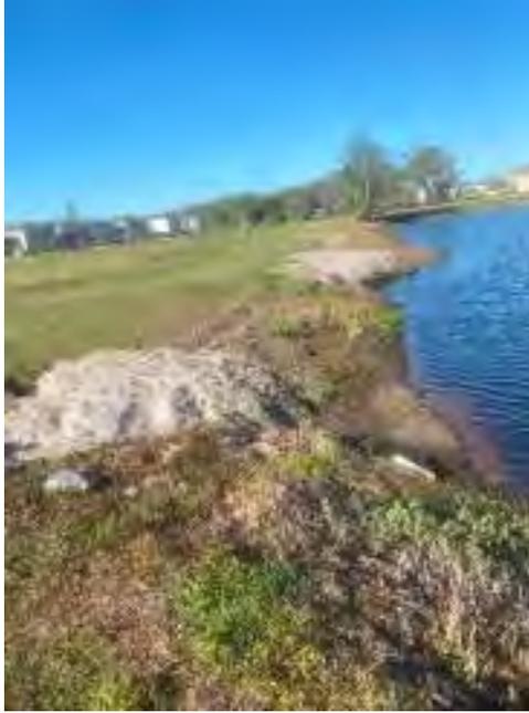
**Location 6:** Broken pipe discharge causing erosion. Remove back to first joint and replace to outfall at pond toe of slope. Install rip rap at outfall of pipe. Sod all disturbed areas.
