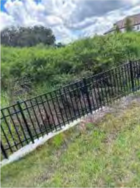
**Location 10:** Overgrown vegetation needs to be cleared 5' from headwall to allow proper flow and discharge into and from drainage pipes.
