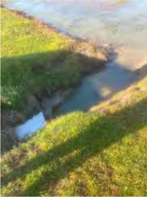
**Location 7:** Existing mitered end section is undermining on discharge side. Add sand cement bags to end of mitered end section discharge to match the mitered end section outfall elevation. Sand cement bags are not to be installed above the mitered end section restricting flow.
